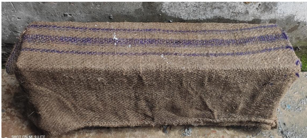
Figure 22: Beam curing
