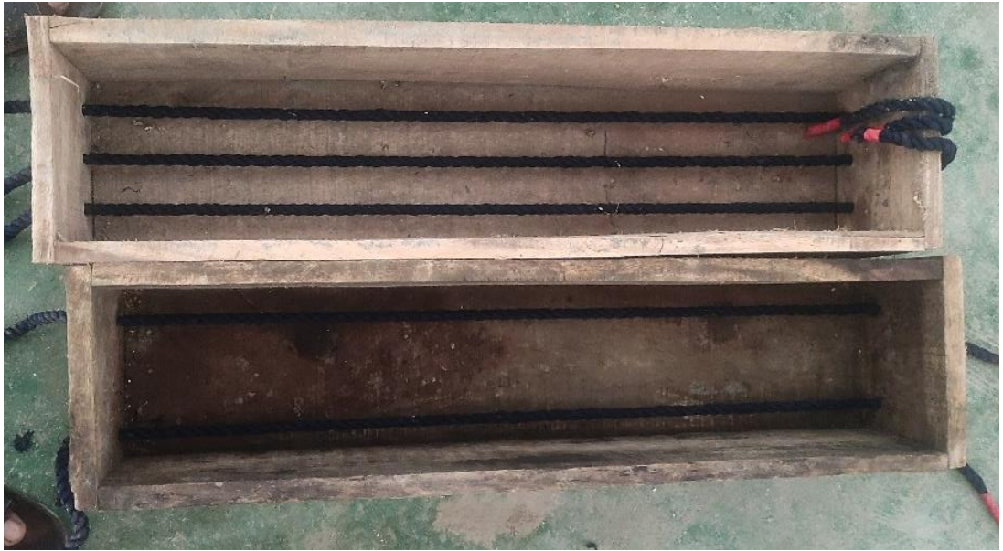
Figure 19: Formwork setup
