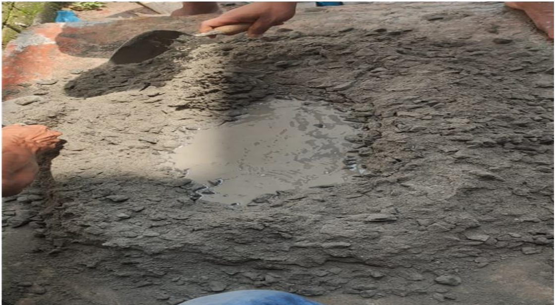
Figure 8: Manual mixing of concrete
