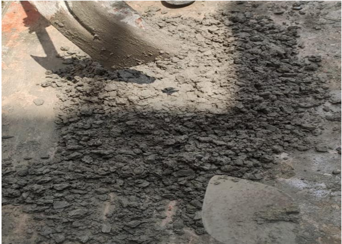
Figure 9: Wet concrete mix
