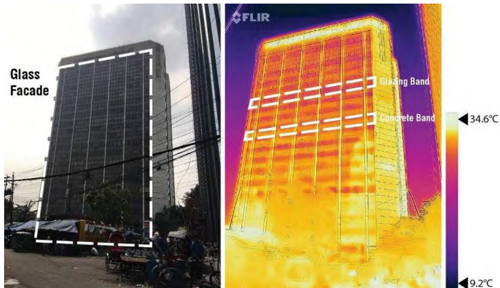
Figure 4.4: Investigation of the streetside facade of SKB.
