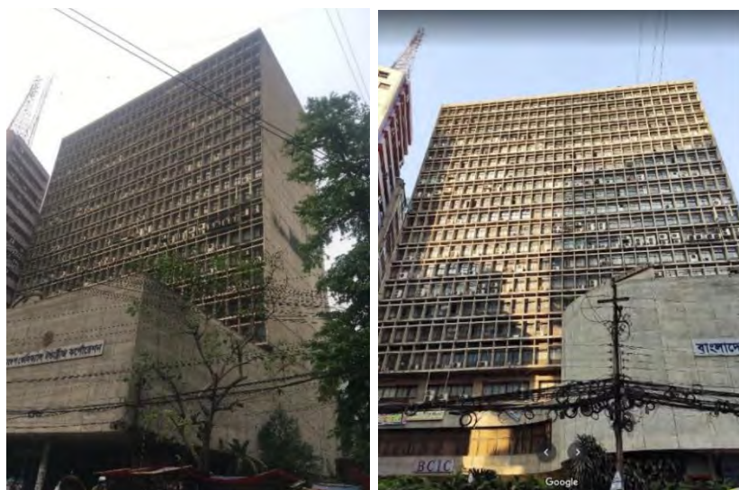
Figure 4.10: Street views of BCIC Building.
