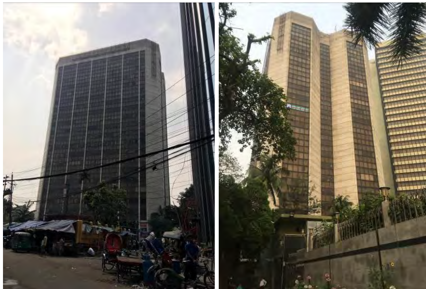
Figure 4.16: Street views of SKB.
