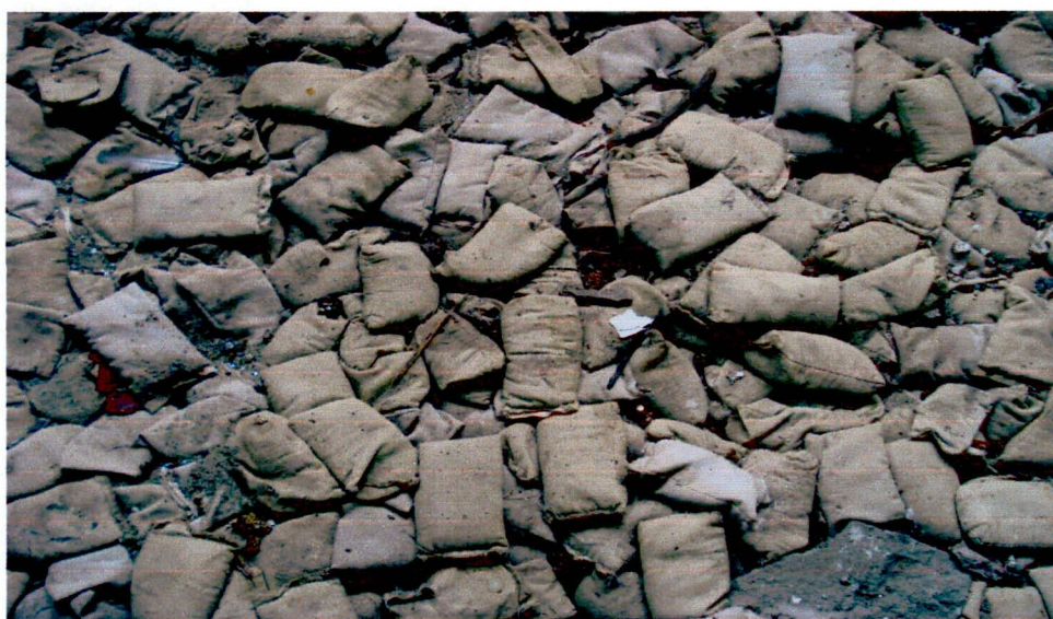
Figure 3.5 Preparation of Geobags (Grade 4, length 17 mm, width 13 mm)
