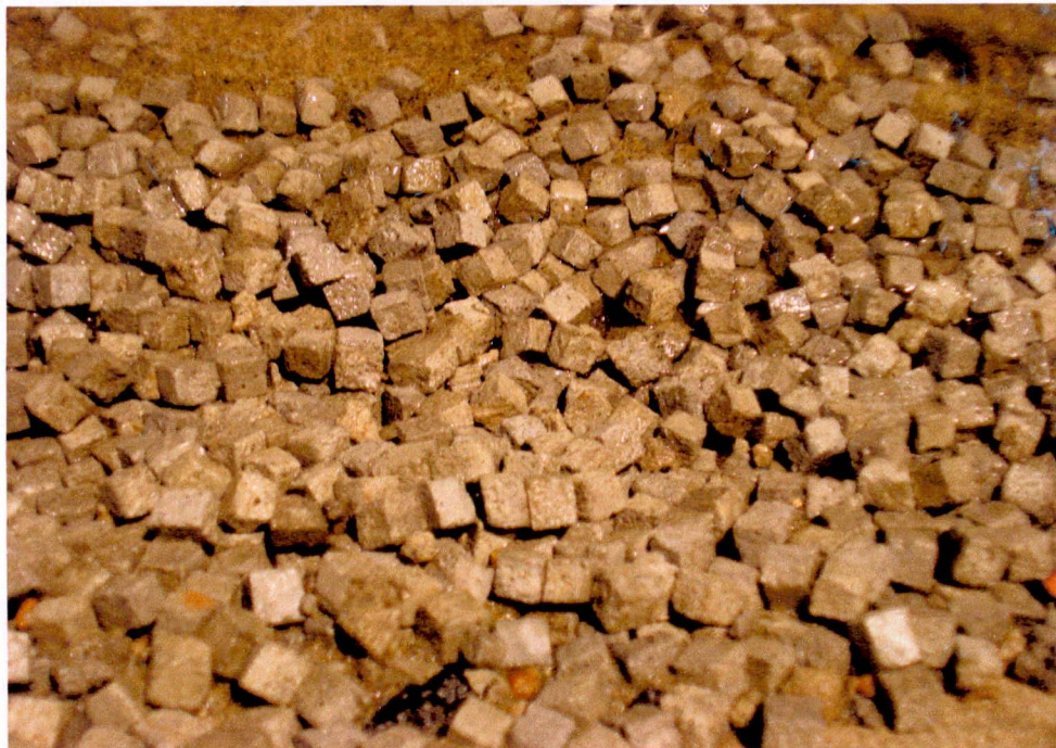
Figure 4.37 Scour hole around 3mm apron
