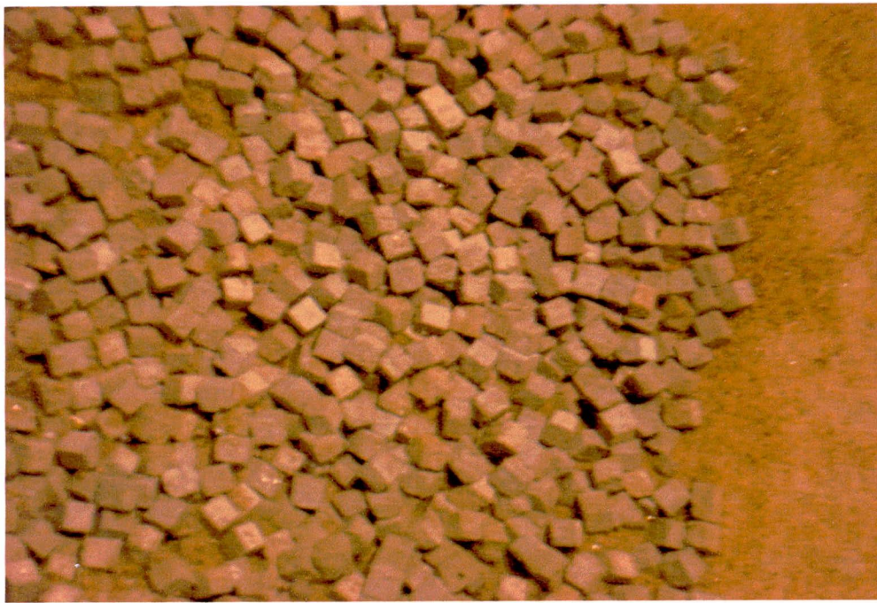
Figure 4.38 Launching of apron to prevent scour
