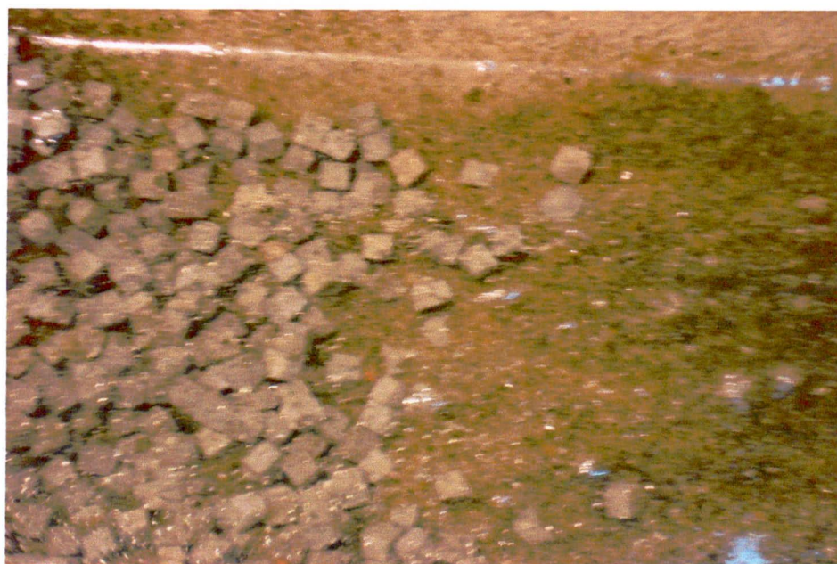
Figure 4.21 Launching of 3mm apron
