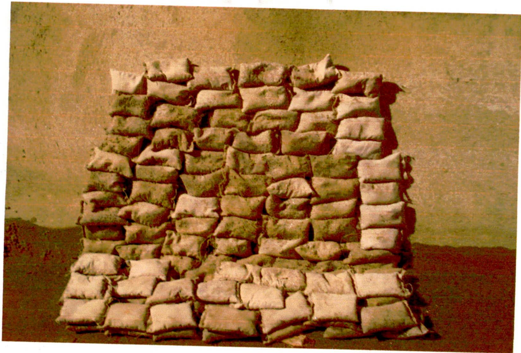
Figure 3.12 Placement of Blocks at the toe of the revetment
