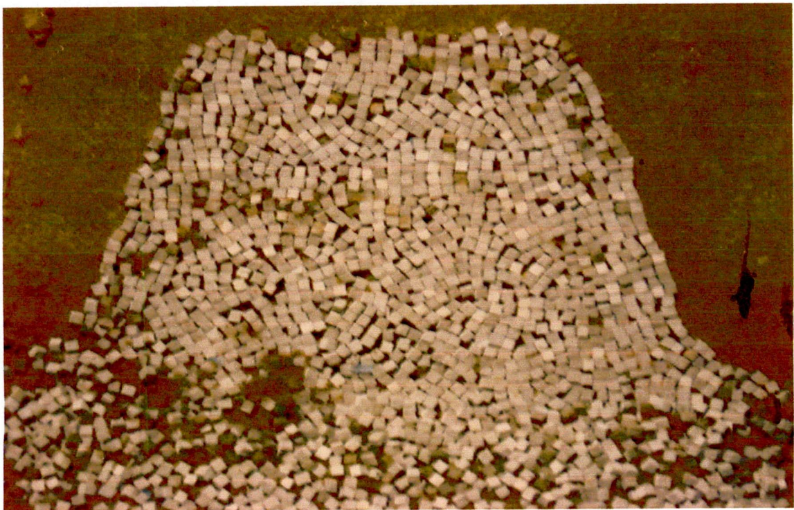
Figure 3.11 Placement of Blocks at the toe of the revetment
