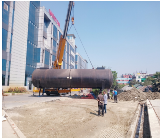
Figure:01;The picture of cyclopentane C5 chemical underground storage tank.
