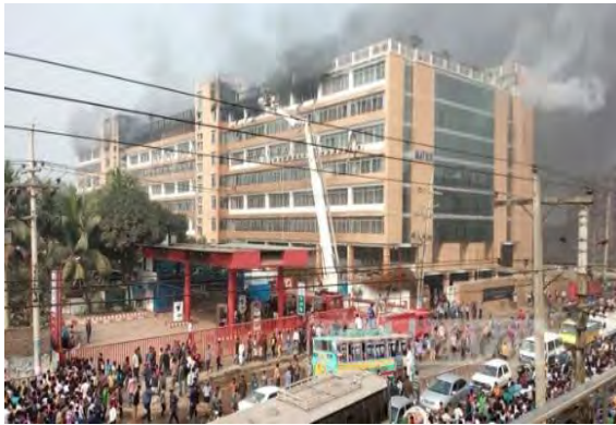
a) Eight-storied factory building of Matrix Sweater Ltd, Gazipur, 2/2/2016,
