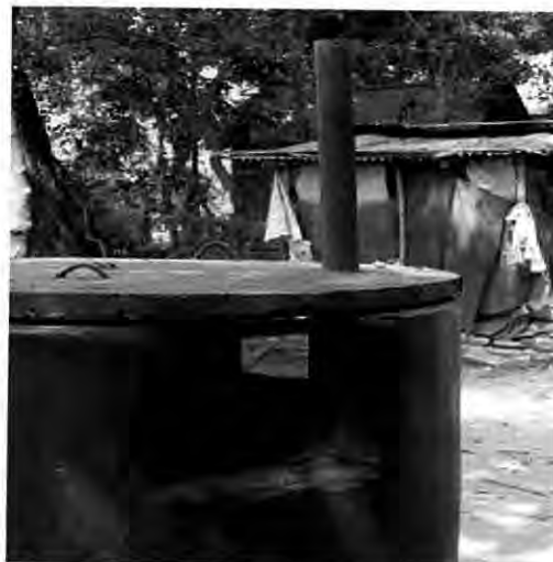
Fig. 2.5: Dug Well with Removable Concrete Cover
