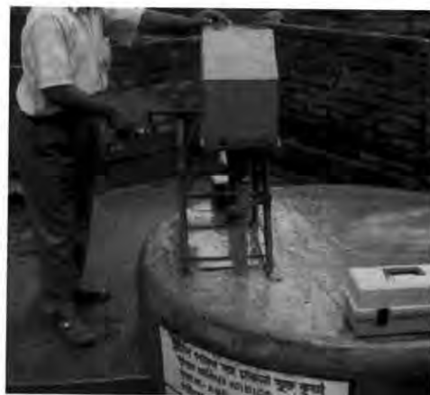
Fig. 2.9: Dug well with Row pump
