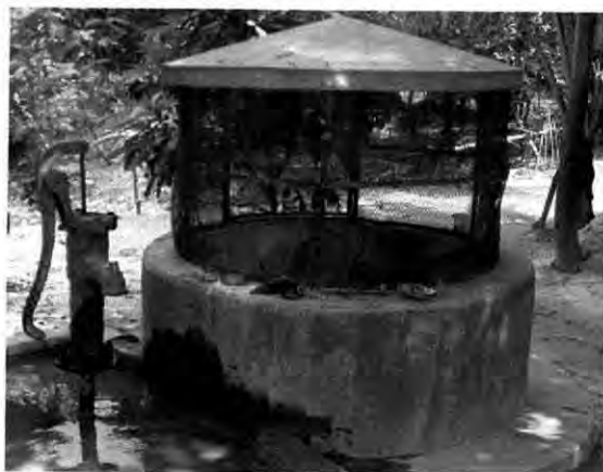
Fig. 2.7: An Improved Dug Well
