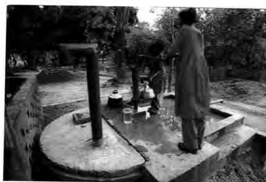
Fig. 2.4 : Water Collection from a Closed Dug/Ring Well by Tubewell
