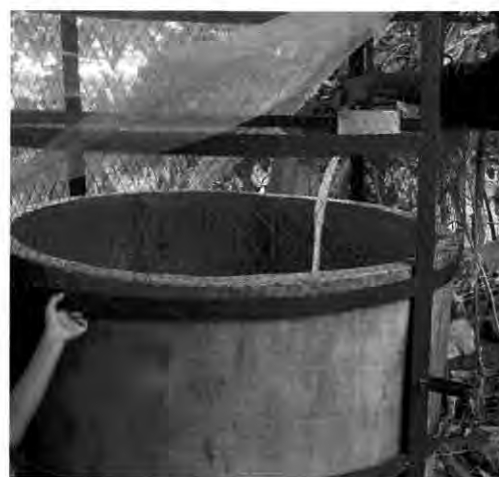
Figure 3.5: Pouring of bleaching powder mixed water into the dug well
