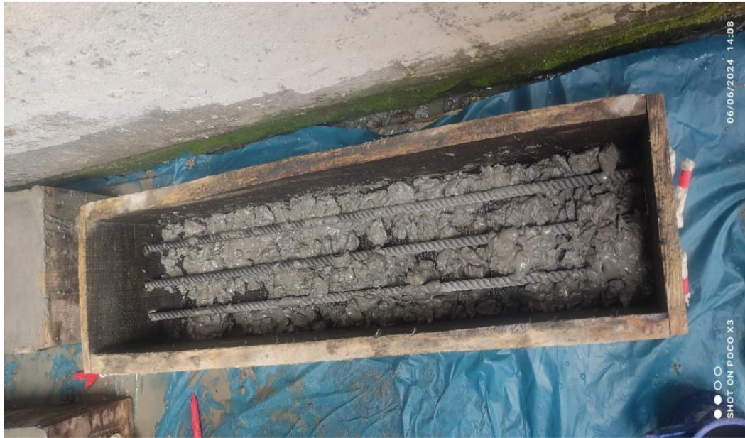
Figure 3-22: NRC Beam Casting
