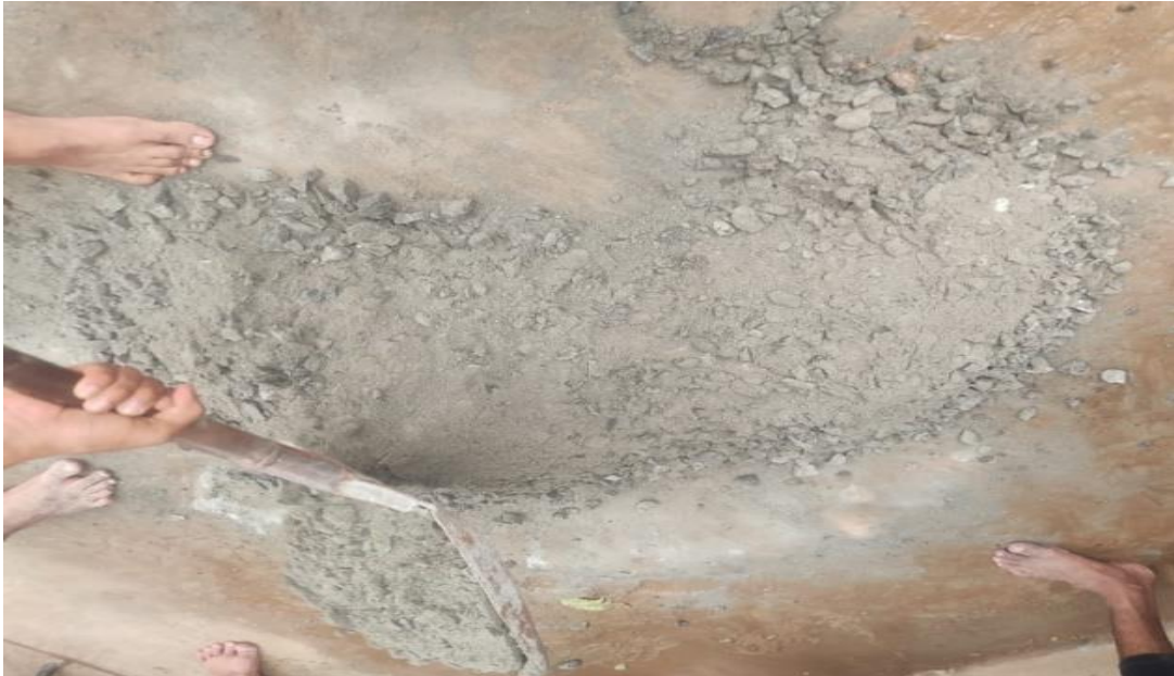
Figure 3-5: Before Concrete Mix
