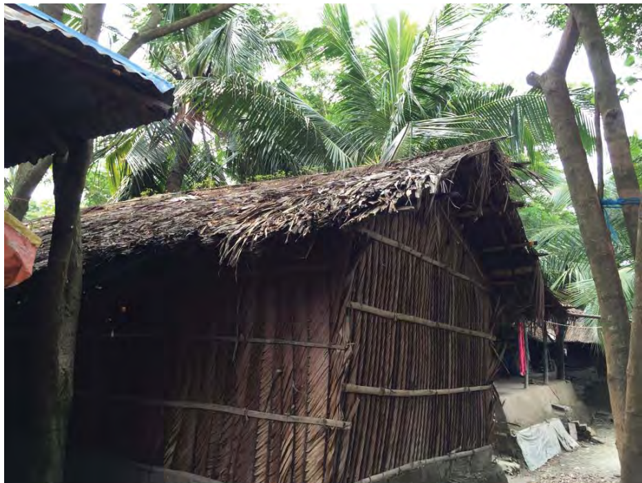
(c) Outside of dwelling unit
