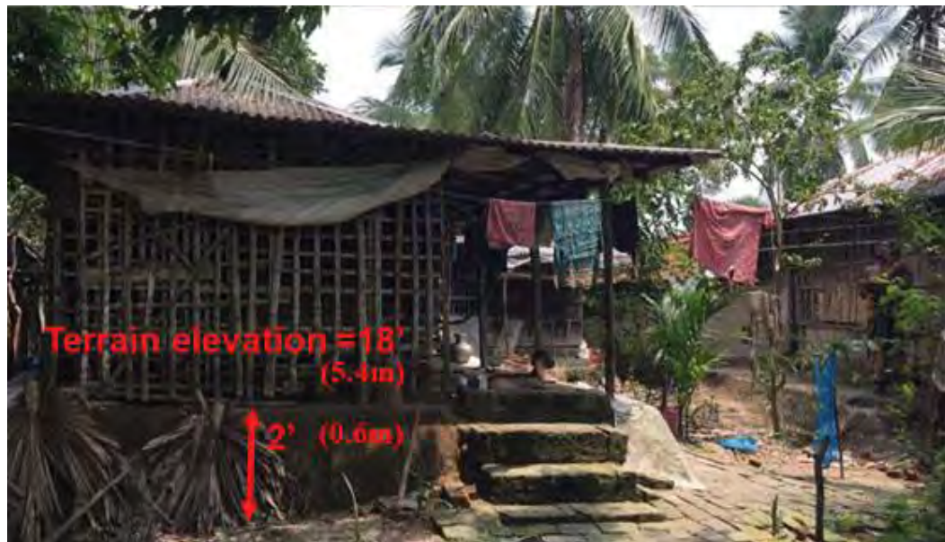
(c) Terrain elevation 5.4m, Plinth 0.6m
