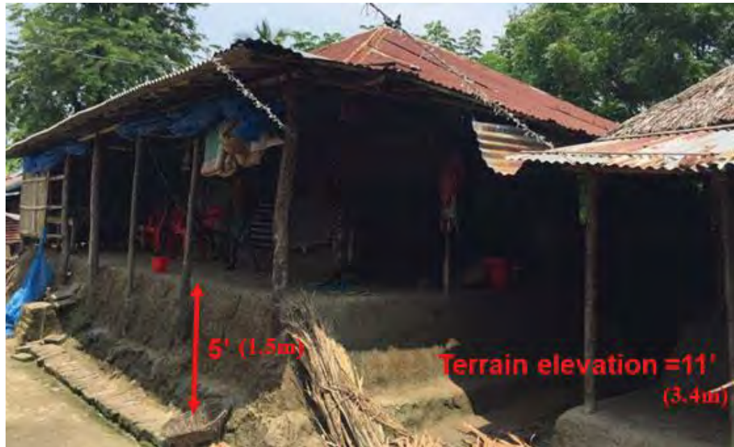
(b) Terrain elevation 3.4m, Plinth level 1.5m
