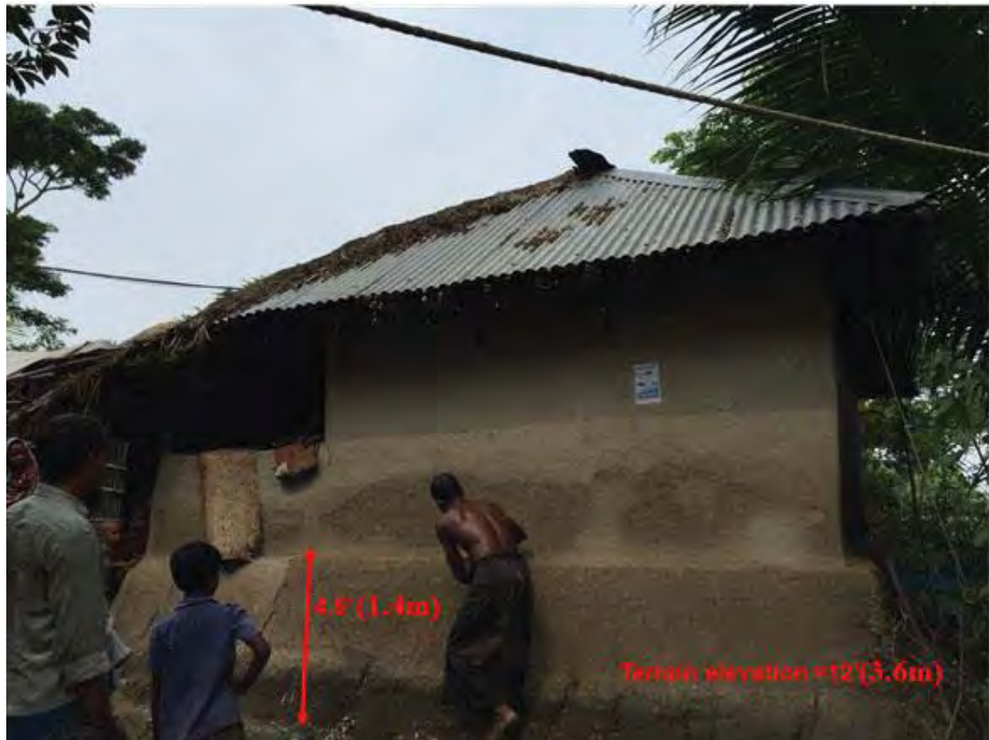
(a) Terrain elevation 3.6m, Plinth level 1.4m
