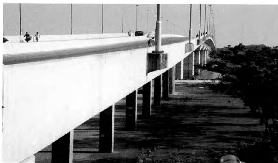
Photograph 5.3: Bridge Sight View from Bhairab End.
