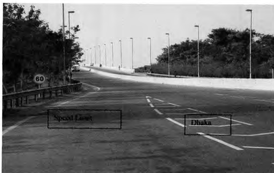
Photograph 5.1: Bangladesh-UK Friendship Bridge from Ashuganj End.
