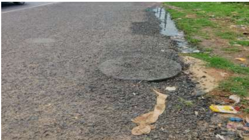
Figure 4.8.4: Manhole Cover Over the Top Surface of Road
