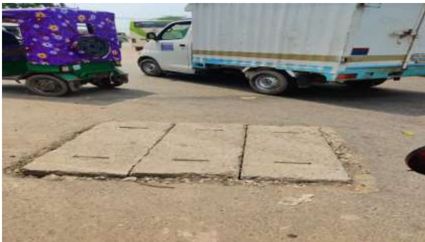
Figure 4.8.2: Drainage Concrete Over the Road
