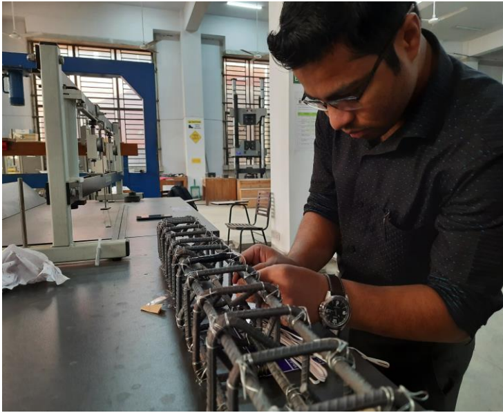
(a) Installation of Strain Gauge on Column Reinforcement
