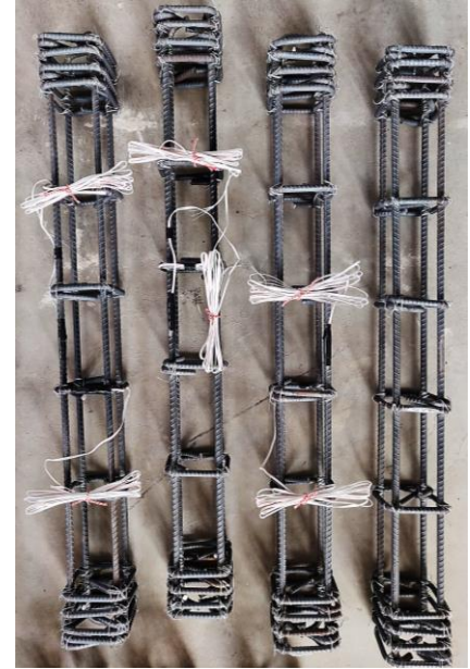
(b) Column Reinforcement Detailing
