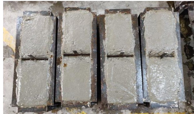
(f) Casting of Beam Specimens
