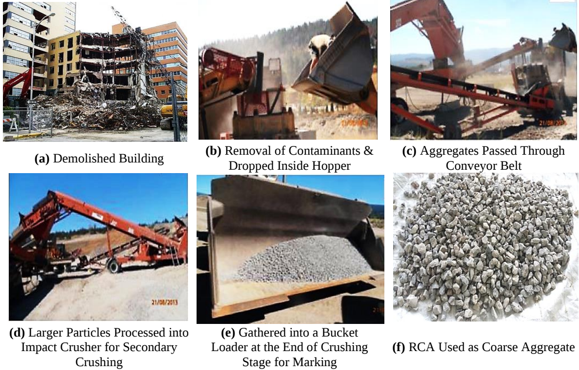
Figure 2.1 Production of RCA (modified images from sources [2, 16, 42]).
