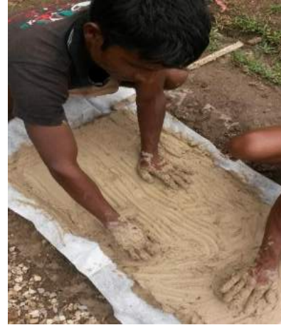
(j) Providing the geo-textile in third row
