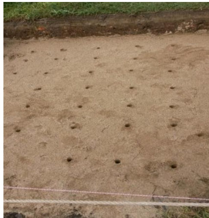
(a) Shear key on compacted bed
