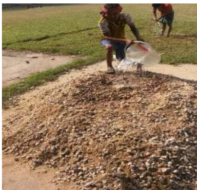
(c) Addition of water
