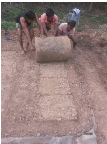
(f) Rolling by one ton concrete roller
