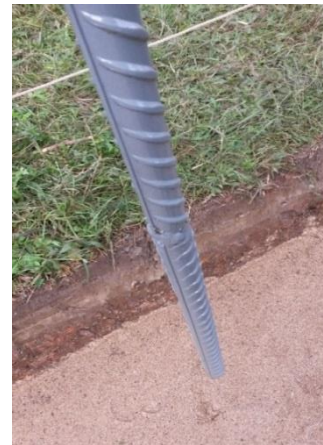
(b) Rebar used to generate shear key
