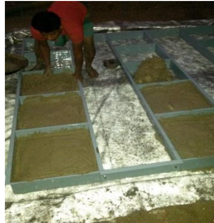
3.25 Casting of bulli inside Steel casing
