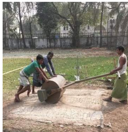
(h) Rolling by two ton steel roller
