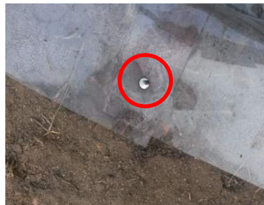
(a) Anchoring of plastic sheet by pin shape nails (in circle)
