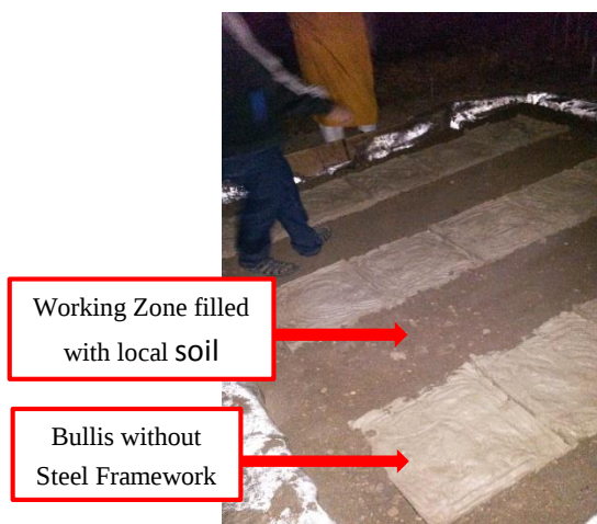
(e) Bulli after 1st stage construction
