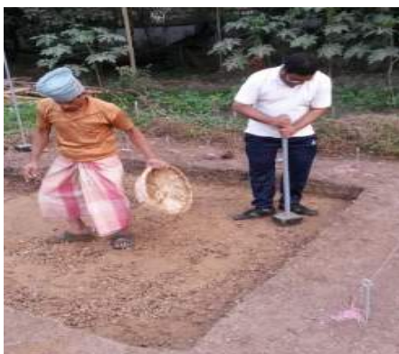
(e) Compaction by hand compaction
