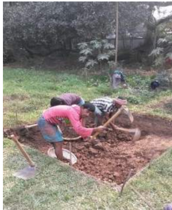
(c) Excavation work
