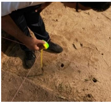
(a) Checking of Reduced Level( RL)
