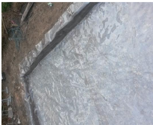
(c) Placement of plastic sheet above base
