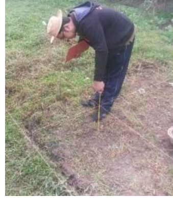
(b) Measuring RL. Of layout line
