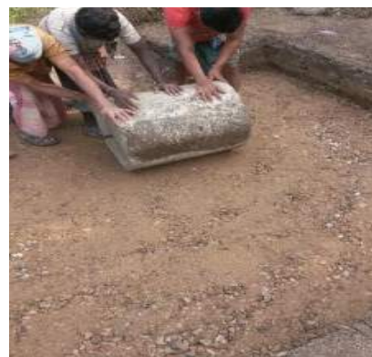
(f) Compaction by manual roller
