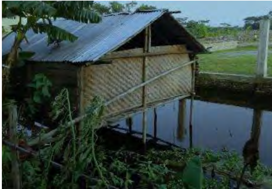
Figure 6.13 Canal Encroachment by Land Invader
