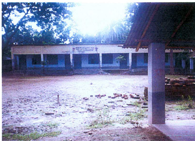
Photo 6 Bheti Camp in Raninagar Thana, Naogaon.
