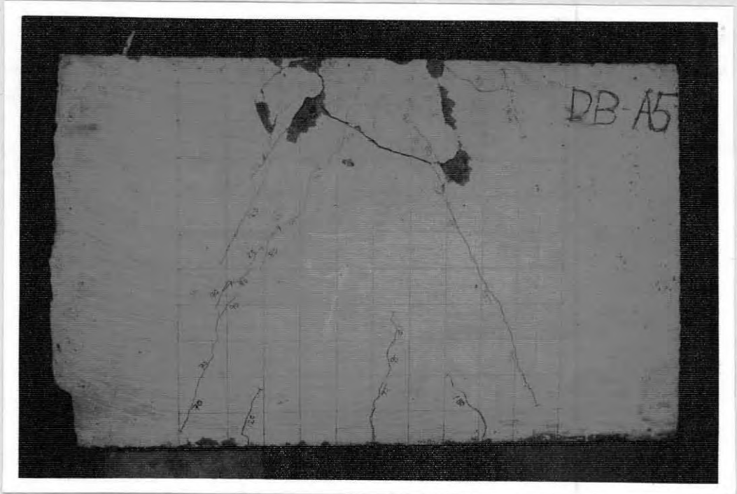
Fig. 5.43 Observed mode of failure and the crack pattern of Beam DB-A5
