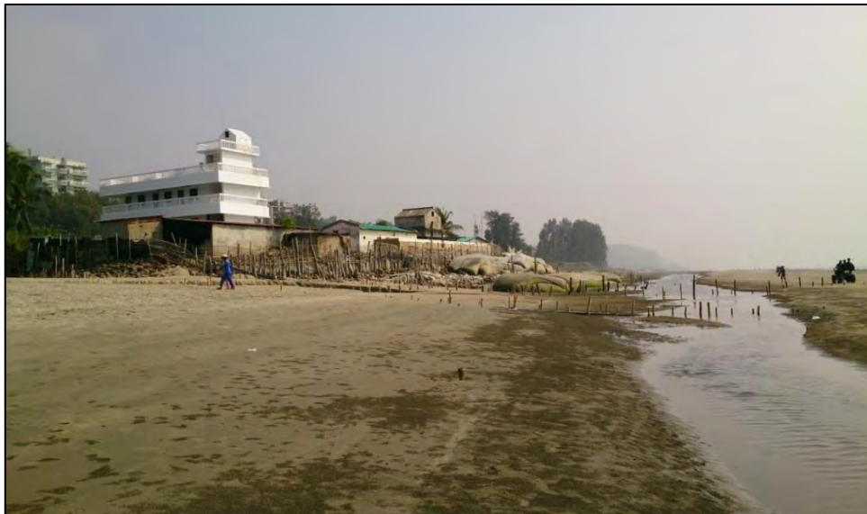
Figure 4.3: Local protection measures due to erosion at Hatcharipara, Cox-Bazar
