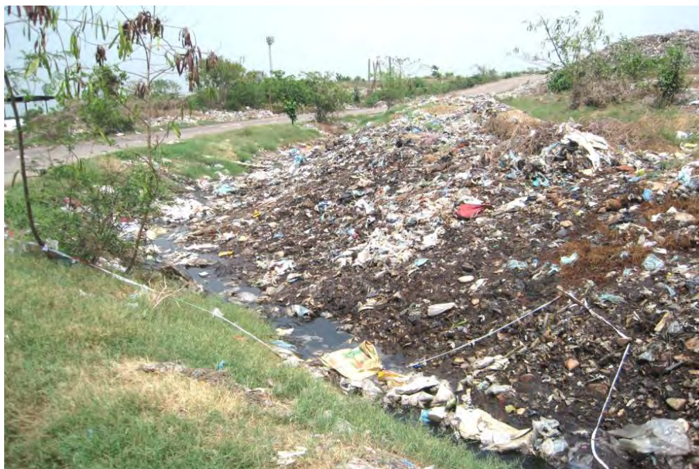
Photograph-A9: Drainage System at Matuail Landfill Site under DSCC was observed during Field Survey in April, 2013
