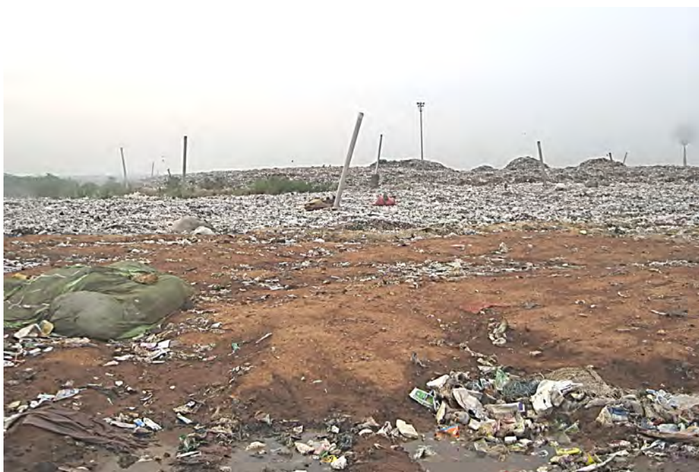
Photograph-A11: Gas vent Pipe using for Landfill Operation was found during Field Survey in April, 2013 at Amin Bazar Landfill Site under DNCC
