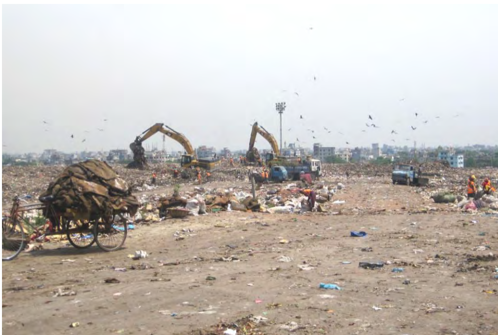
Photograph-A7: Excavator is using for Landfill Operation was observed during Field Survey in April, 2013 at Matuail Landfill Site under DSCC
