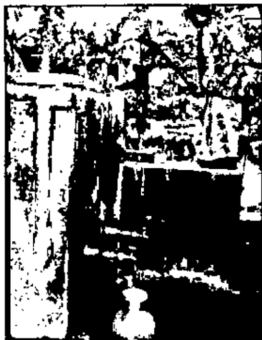
13. An Active Pond Sand Filter
