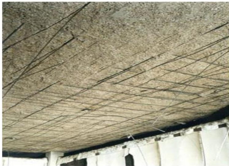
Figure-2.14: Effect of Fire on the Ceiling [10]
