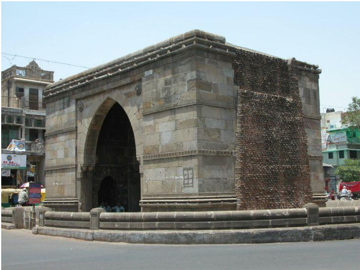
Figure 50: Current view of Astodia Gate showing severed edge of the 'Wall'
