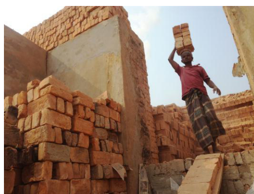
Plate 12: Unloading brick from brick field chamber
