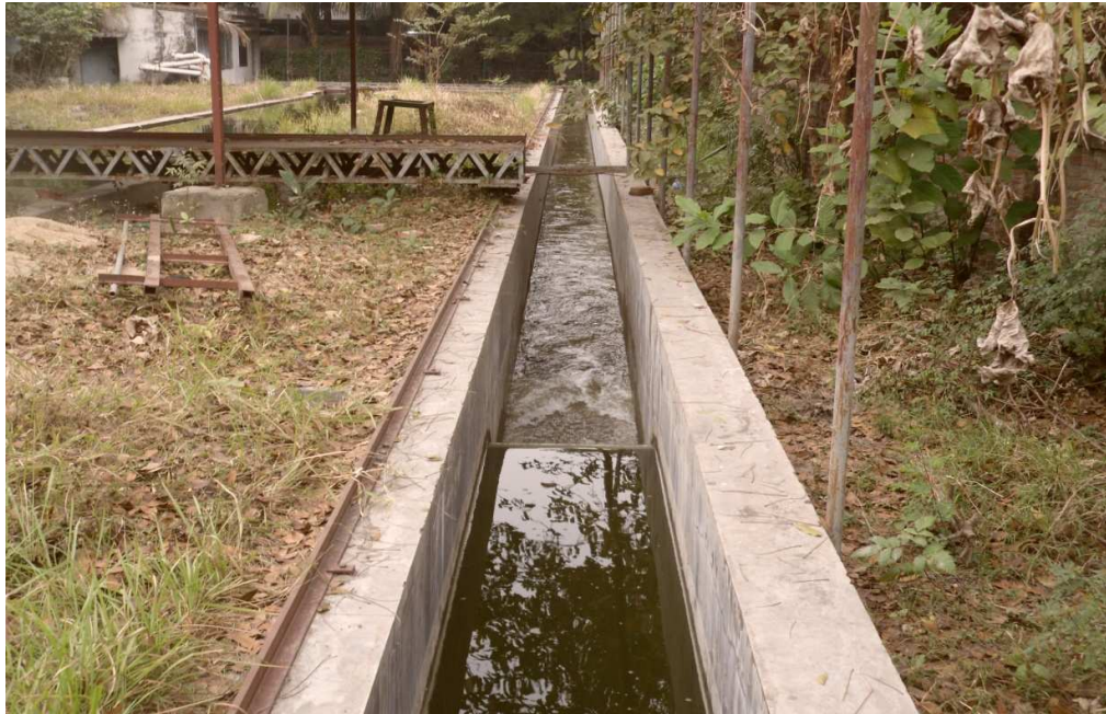
Photo D-9: The Transition Flume
