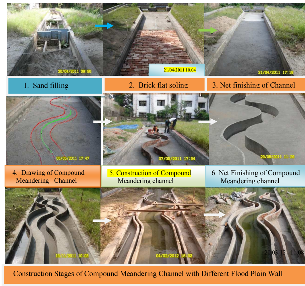
Figure 3.5: Construction Stage of Compound Meandering Channel
