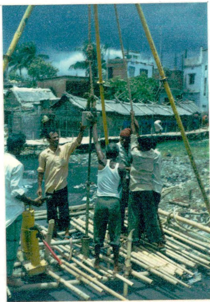
Figure 4.5 Photographs showing boring operation in the tannery wastewater disposal area at Hazaribagh (BH-1)
