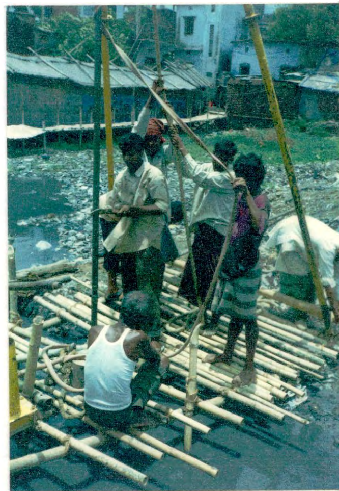
Figure 4.5 Photographs showing boring operation in the tannery wastewater disposal area at Hazaribagh (BH-1)
