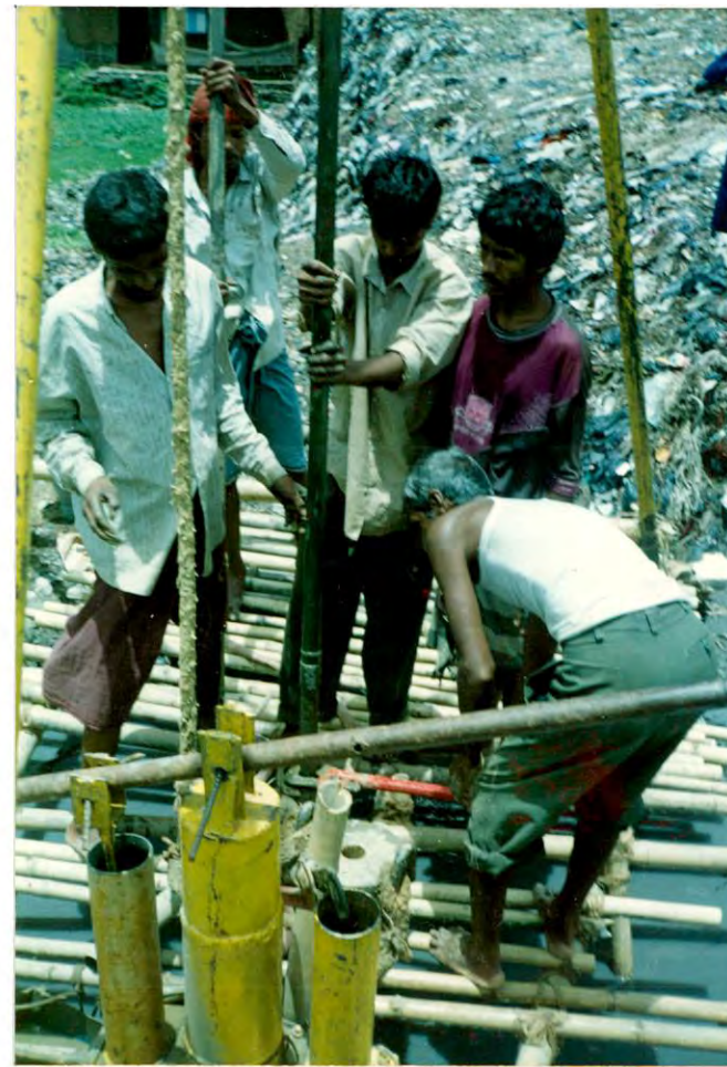
Figure 4.4 Photographs showing boring operation in the tannery wastewater disposal area at Hazaribagh (BH-1)
