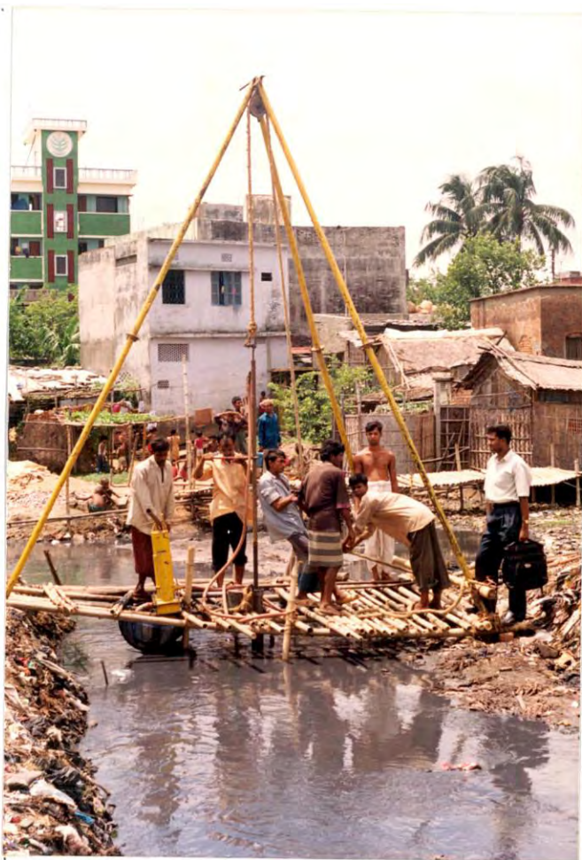
Figure 4.4 Photographs showing boring operation in the tannery wastewater disposal area at Hazaribagh (BH-1)
