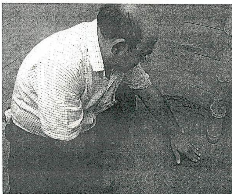
Figure 4.2: Check of compactness of CCL
