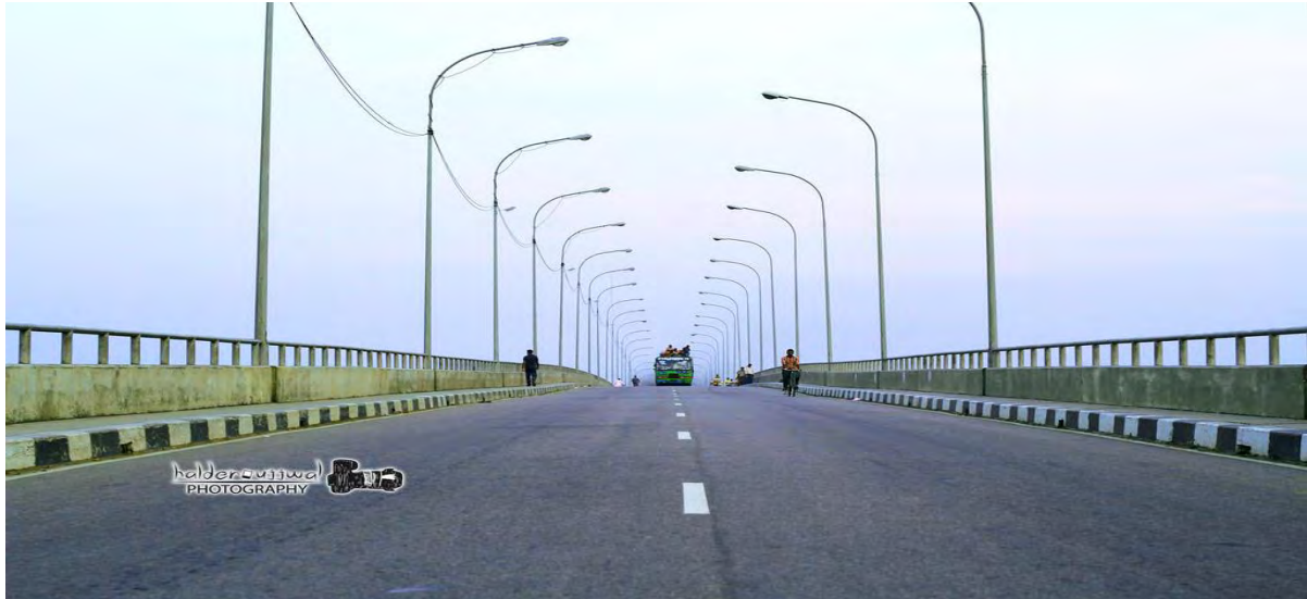
Figure 6.11: Recently Built Dapdapia Bridge at Barisal That Connects the Other Side of Kirtonkhola River with Barisal City. (Source: Collected)
