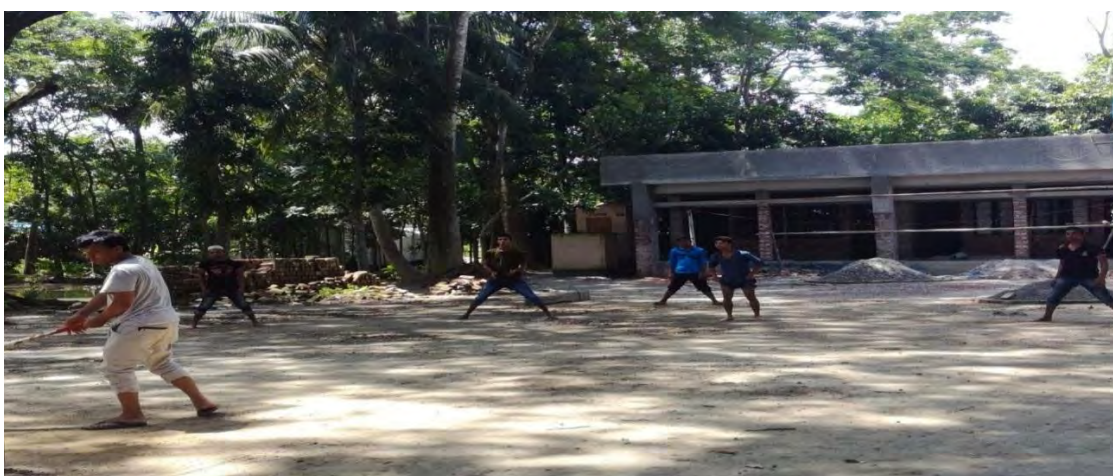
Figure 6.13: Construction of New Academic Building at Batna Government Primary School in Barisal Sadar Upazila
