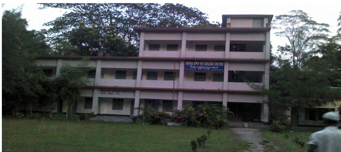
Figure 6.14: Academic Building of Abdur Rashid Khan High School in Char Kowa in Barisal Sadar Upazila
