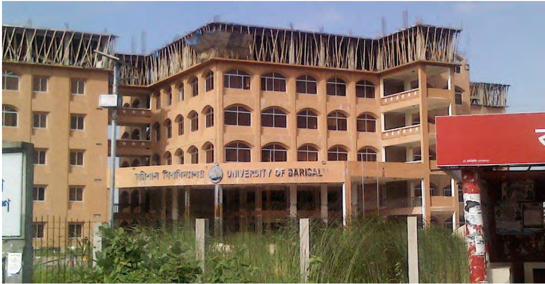
Figure 6.15: Construction of Barisal University in Barisal Sadar Upazila
