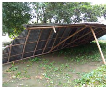
7. f) House construction material salvage
