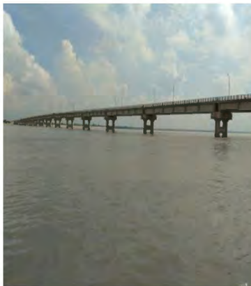
5. b) Mohipur bridge in Teesta
