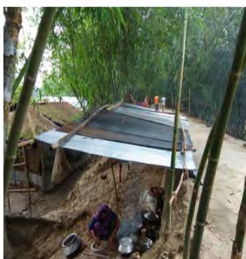
7. d) Shelter in embankment
