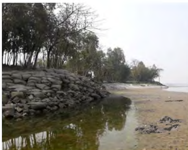
8. d) Erosion protection through sand bag
