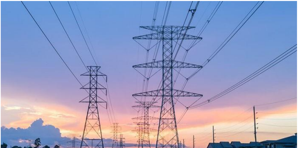
Figure 1.1: Overhead transmission line
