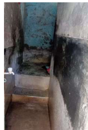
Figure 6.1: Elevated toilet platform in Ceramic Basti by DSK Source: Field Survey, 2022
