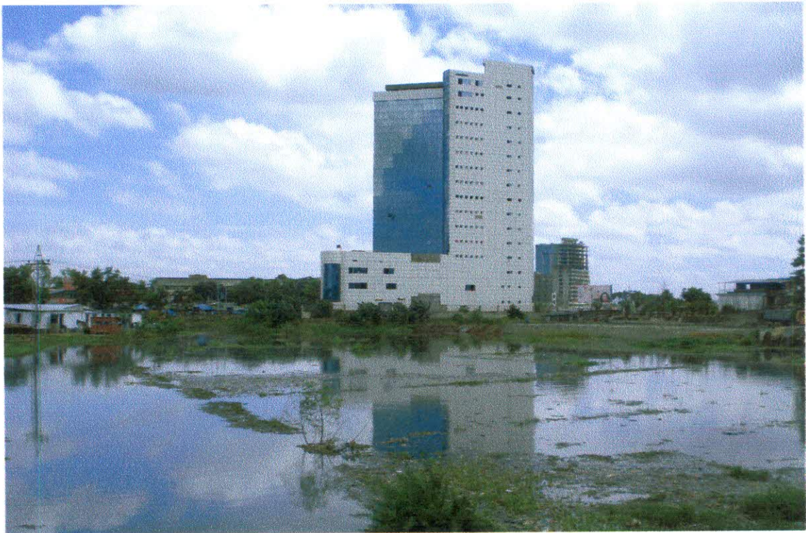
Photograph 7.1 BGMEA building on Begunbari Khal
