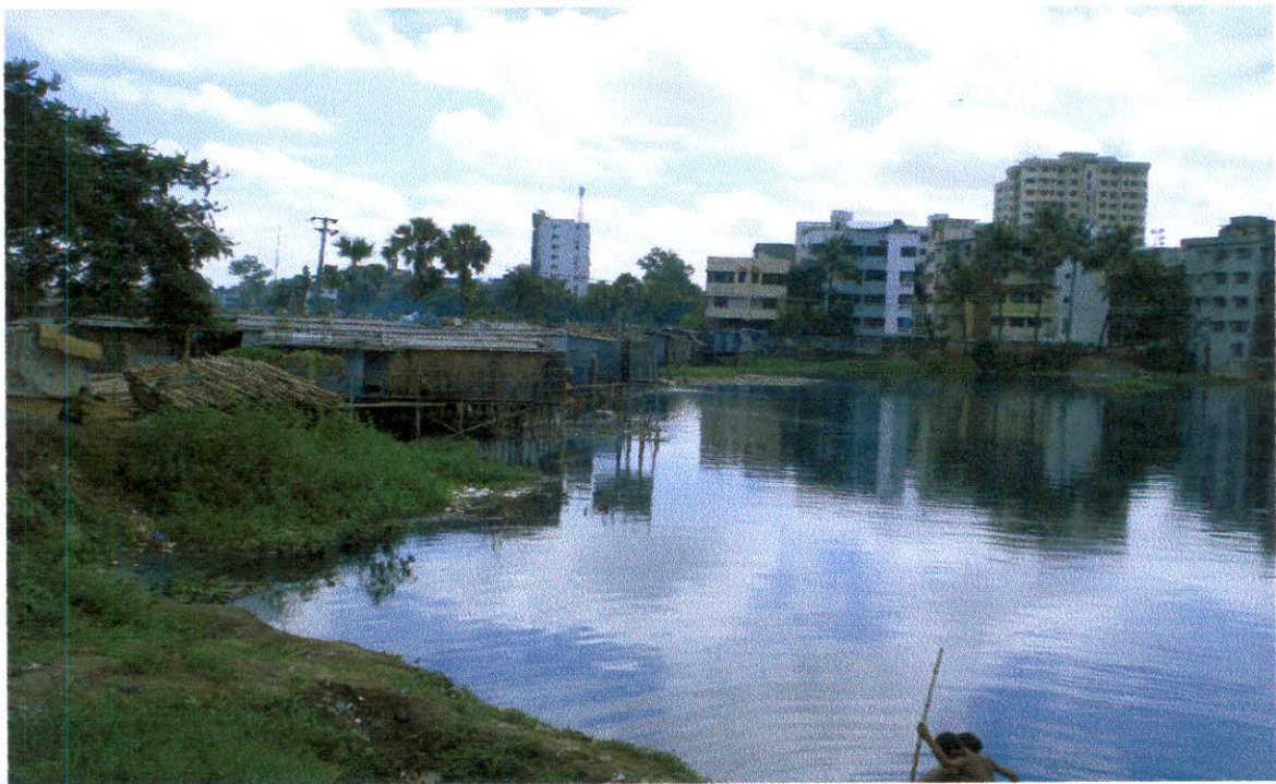
Photograph 5.1 Encroachment of Begunbari Khal by slums
