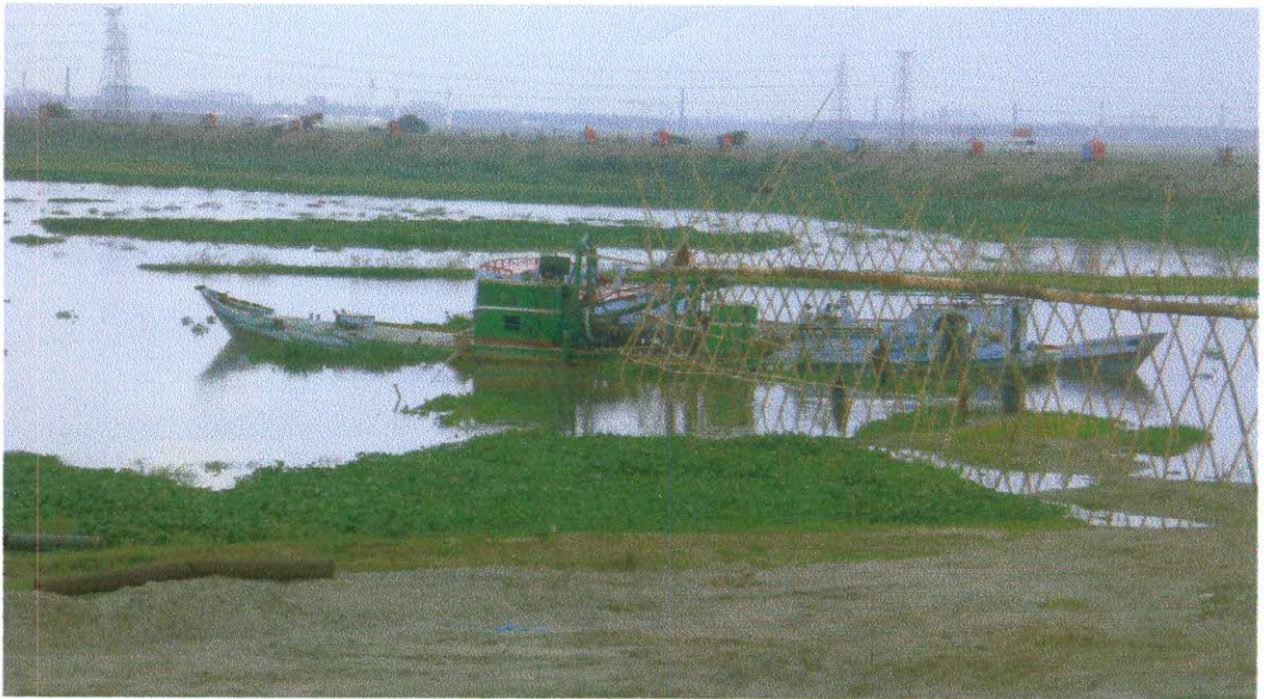
Photograph 8 Dredger are used to fill up the lowland
