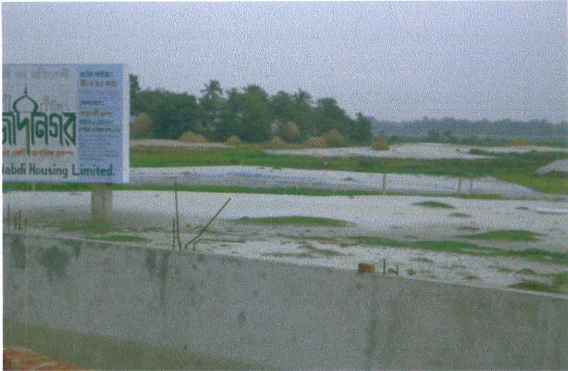
Photograph 4.1 Land filling besides the Balu River
