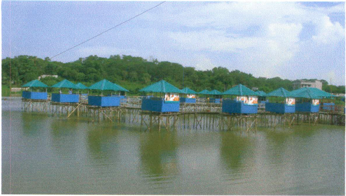
Photograph 7 Unauthorized structures in the wetlands beside the river Turag
