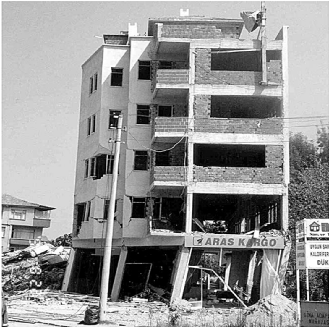
Figure 2.5: Formation of soft storey, Kocaeli earthquake, Turkey, 1999
