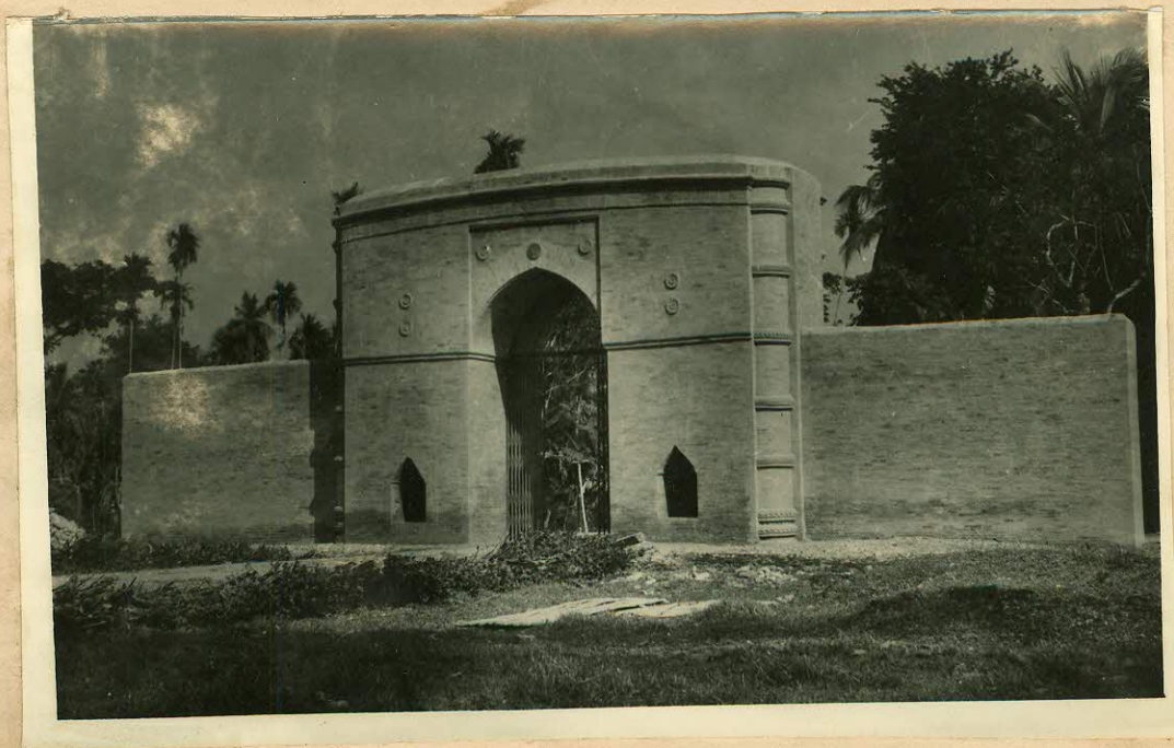
Fig. 1. THE SHĀṬ-GUMBAD MOSQUE, BĀGERHĀṬ : GENERAL VIEW OF THE GATEWAY FROM THE WEST (AFTER RESTORATION).
