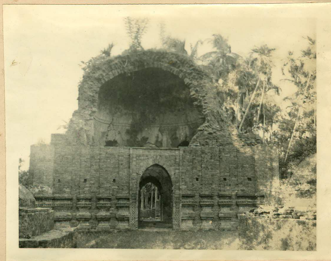
Fig. 2. THE MOSQUE OF ZINDĀ PĪR, BĀGERHĀT : GENERAL VIEW FROM THE SOUTH.
