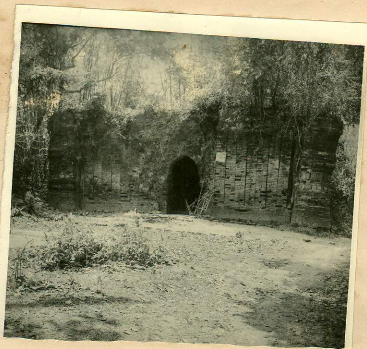
Fig. 2. THE SUVARĀRĀ MOSQUE, JESSORE : GENERAL VIEW FROM THE EAST.
