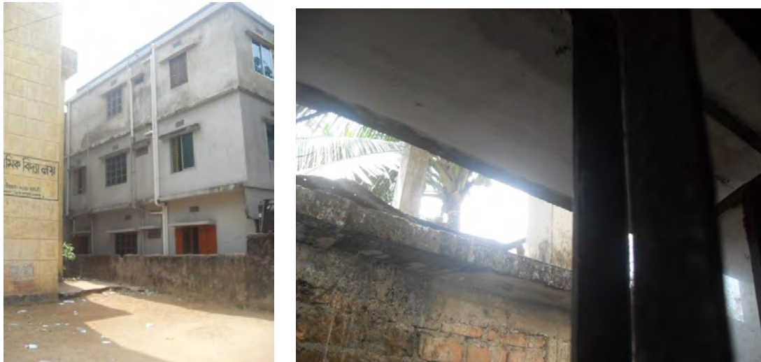
Figure 3.33 Surrounding structures near school building. (Source: Field Survey)
