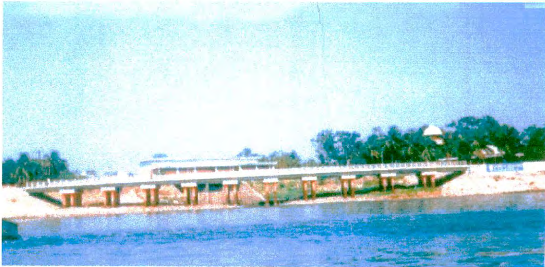
Figure B-1: Dholai khal out fall contains sewage and polluted water
