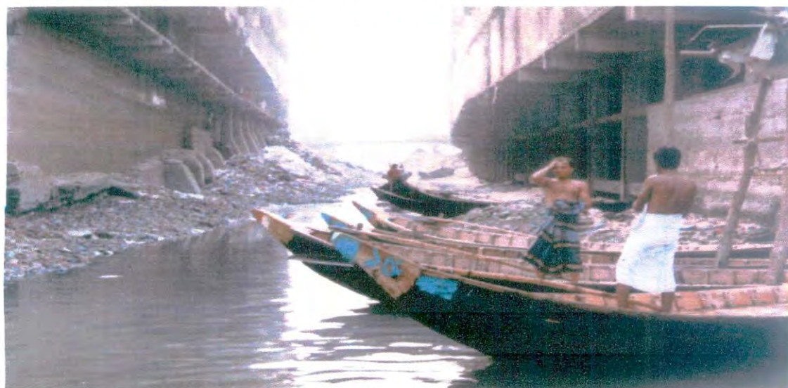
Figure B-11: Industrial effluent discharge point at Kaliganj Bazar
