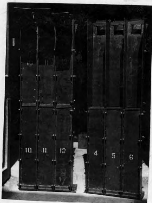
Fig. 4.4 - Formwork for vertical casting of square columns.
