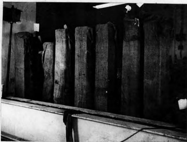
Fig. 4.9-Curing of columns
