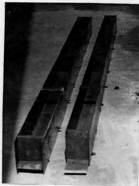
Fig.4.6-Formwork for horizontal casting of square and rectangular column.
