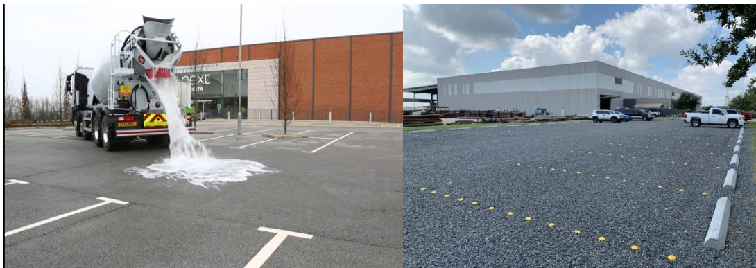
Figure 4-20: Permeable Asphalt Paving Systems (TRUEGRID Paver, USA)
