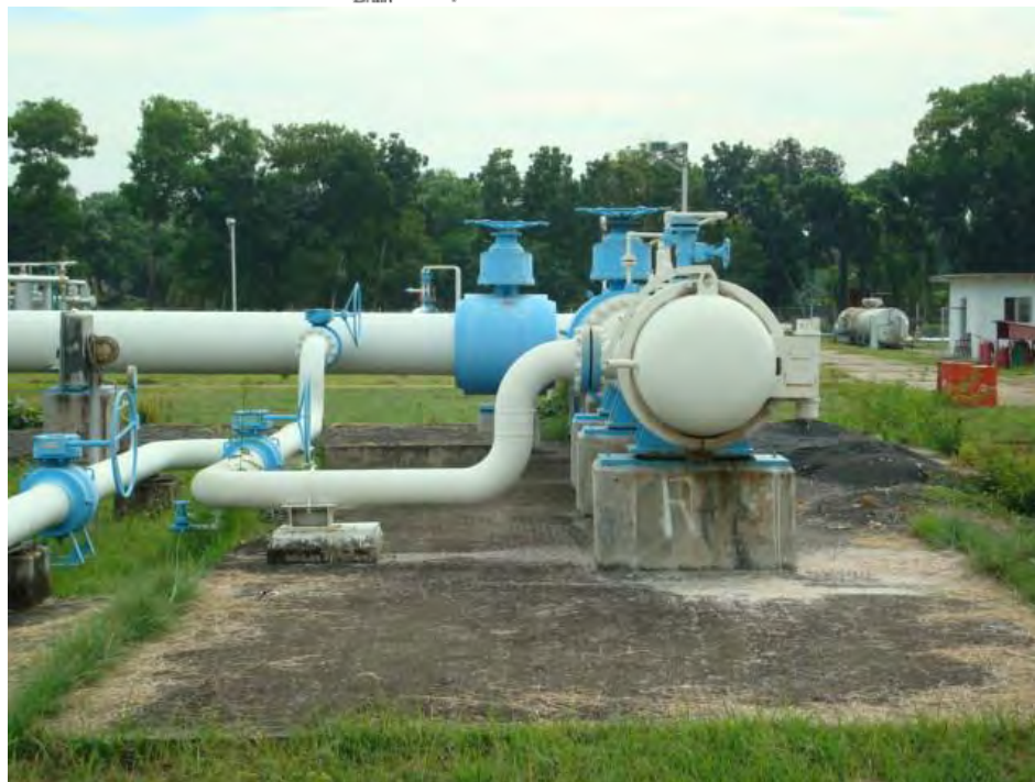
Fig.-A.24: Typical Pig Launcher
