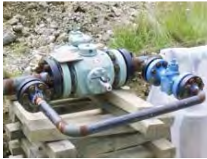
6" Pig Launching Valve being installed with bypass loop.
