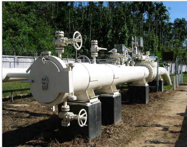
Fig.-A.25: Typical Pig Receiver
