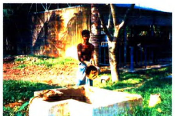
Plate-12 : Concrete Chamber of Bio-gas plant
