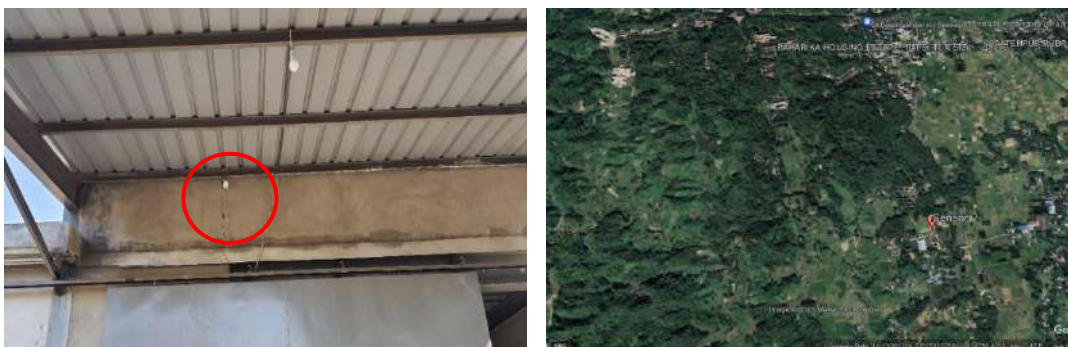
Figure 3.8: Location of sensor at Hathazari
