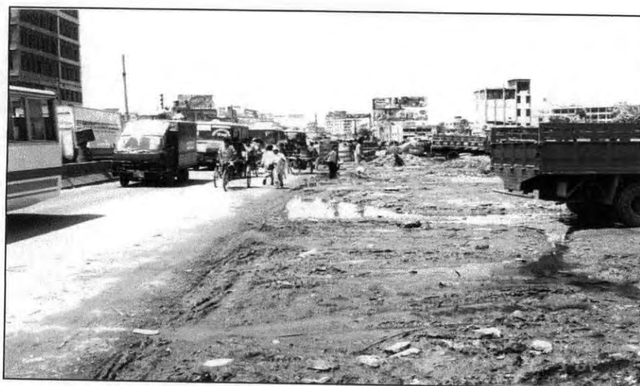
Photo: Water Logged on the Shoulder at Jatrabari
