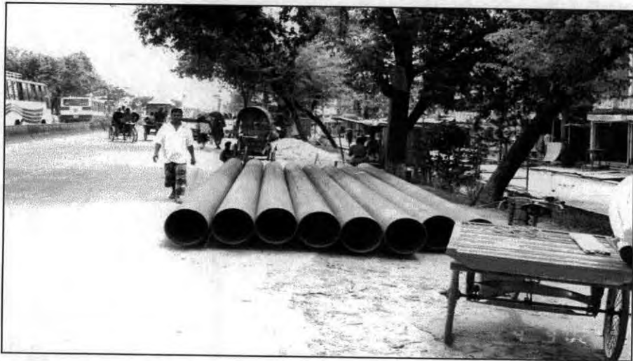
Photo: Gas Pipes Kept on the Shoulder and Carriageway at Rayerbagh
