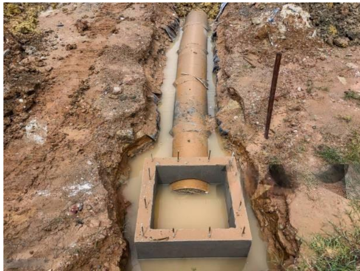
Figure 29 Subsurface drain passing water through the pipe.
