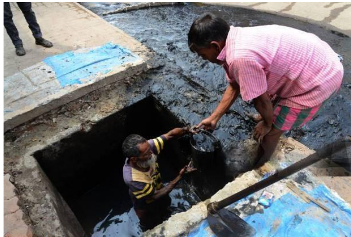
Figure 33 Easy to clean out waste in surface drain
