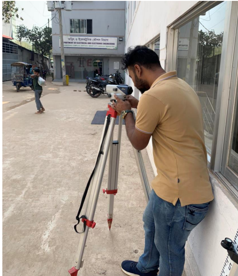
Figure 12 Survey work is going on with 3rd leveling station.
