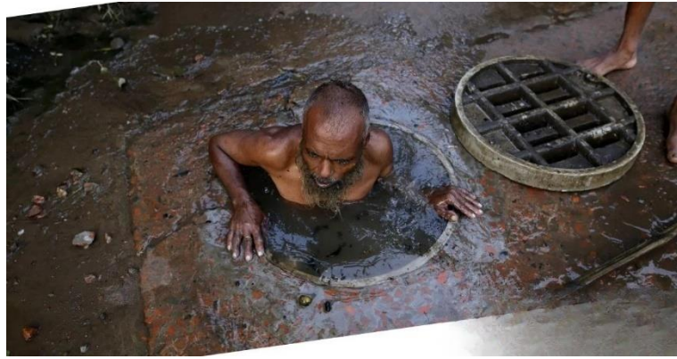
Figure 32 Putting hassle to clean waste in the pipe drain
