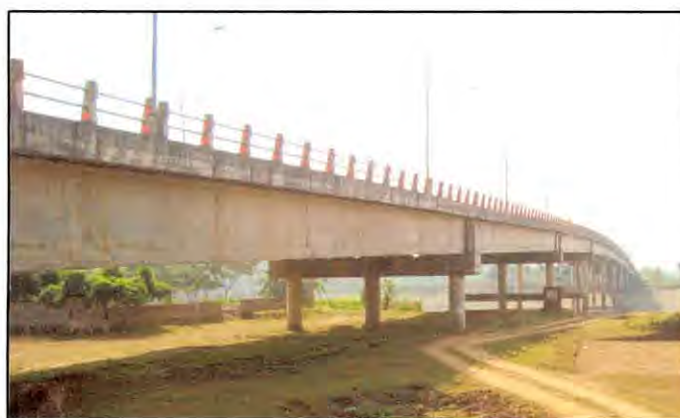
Figure 5.1 Photographic view of Shah Paran Bridge
