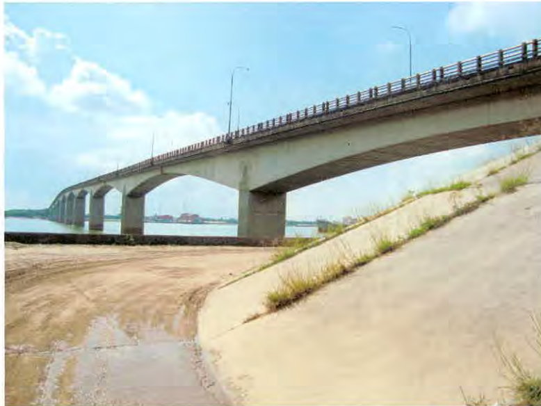
Figure 5.5 Photographic view of Meghna Bridge
