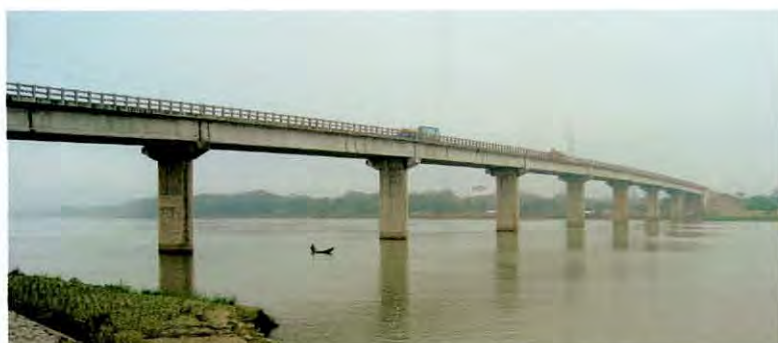
Figure 5.10 Photographic view of Doarika Bridge
