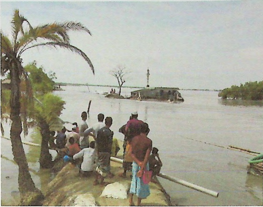
Recently broken the protection dam, Ashashuni, Satkhira, Bangladesh
