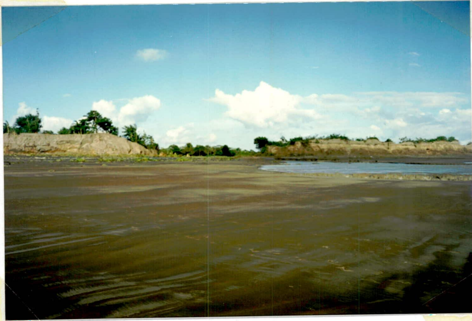
Photo 6: Breach point of old retired embankment near Station 3 at Chainage 4.00 km during low tide (Land side facing)
