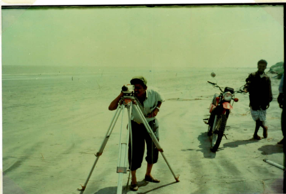
Photo 17: Cross-sectional Survey works across the Beach
