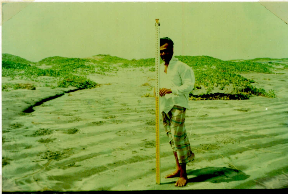
Photo 18: Staff positioning for Cross-sectional survey works across the Beach
