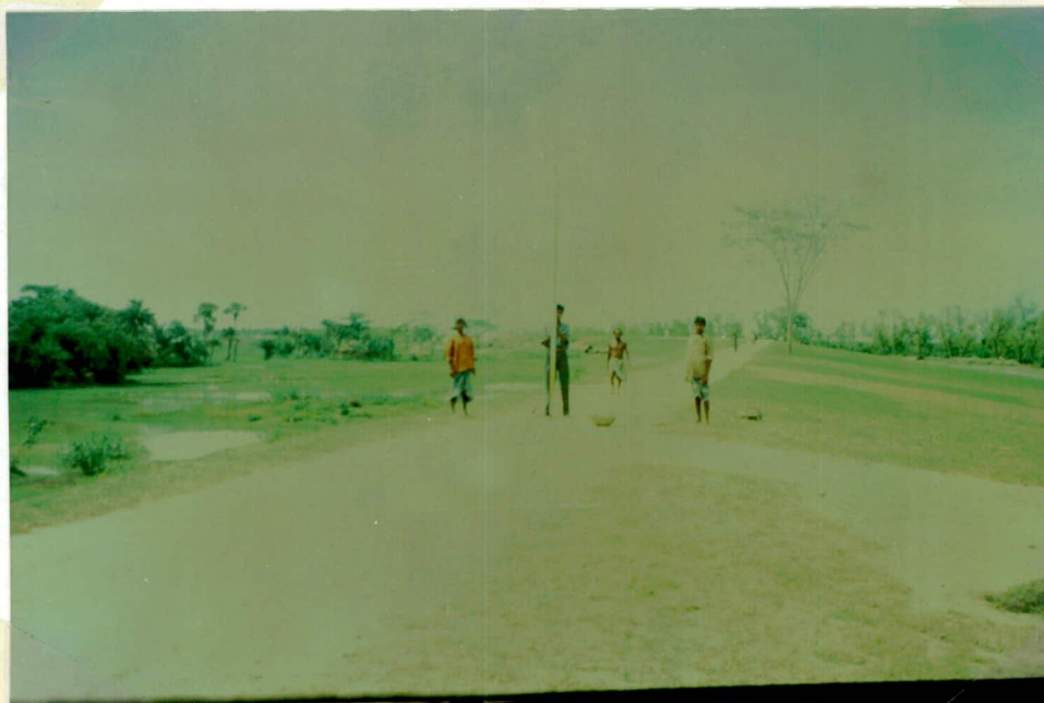
Photo 16: T.B.M. (Temporary Bench Mark) carrying through the Coastal Embankment (Polder No. 48)
