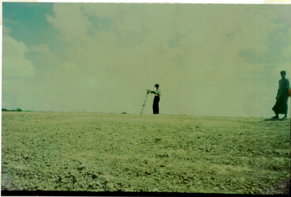
Photo 12: Coastal Embankment (Polder No. 48) at Kuakata (Land side facing)
