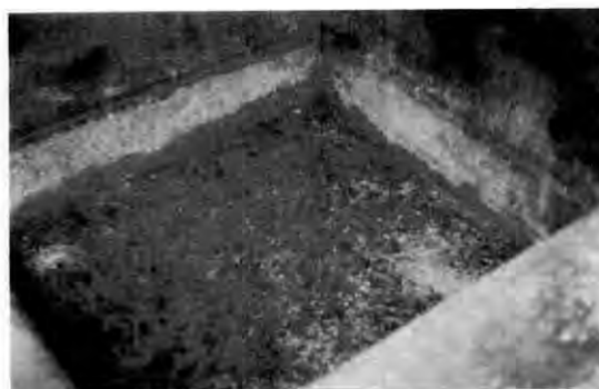
Plate 4.8 Chlorination Tank for Disinfecting Tubes and Plastics
