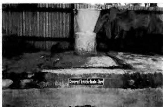
Plate 4.7 Concrete Pit for the Disposal of Syringes, Saline bags and sharps
