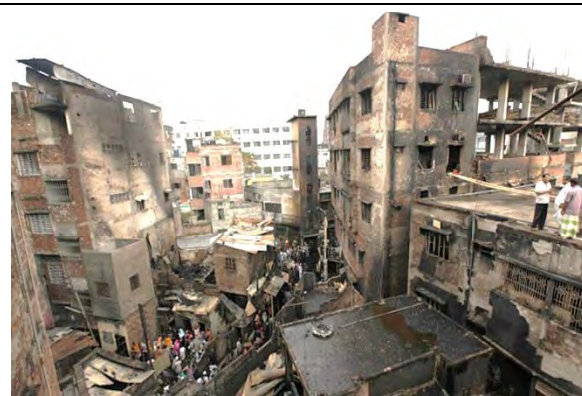
Figure 5-3: Fire Accident of Nimtoli, Old Dhaka (Source: Bangladesh Fire Service, 2010)
