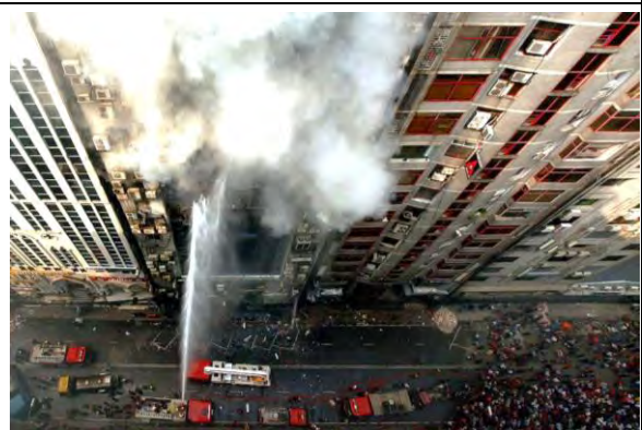
Figure 5-6: Fire Accident of FR Tower, Banani (Source: The Daily Star, 2019)
