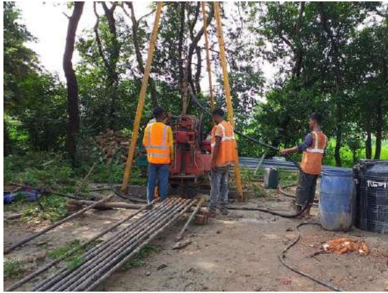
SPT at BH195
