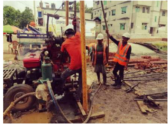
SPT at BH320
