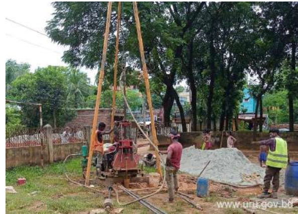
SPT at BH033
