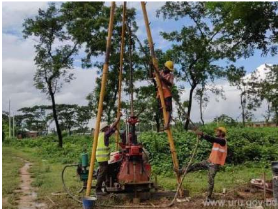
SPT at BH061
