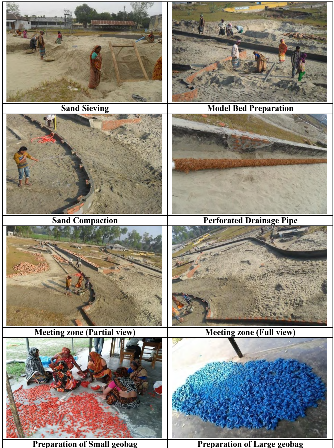
Figure A.2: Pictorial View of Physical Model Setup Construction at Field
