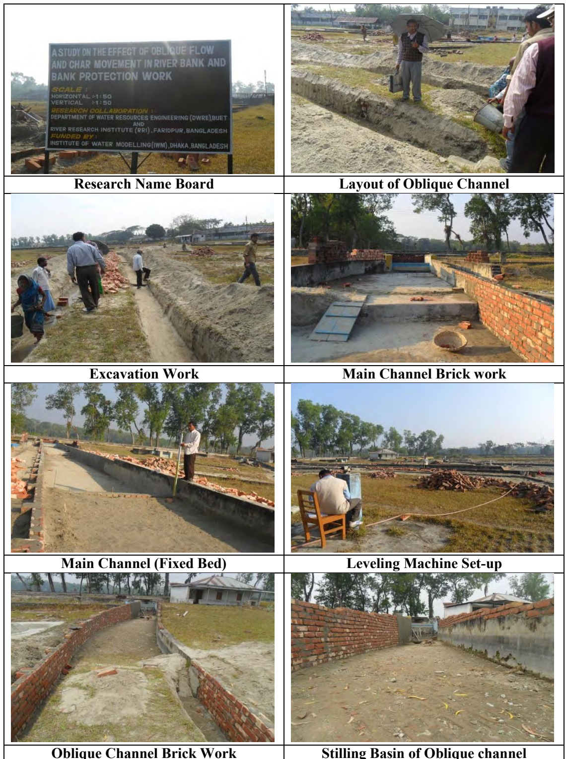
Figure A.1: Pictorial View of Physical Model Setup Construction at Field
