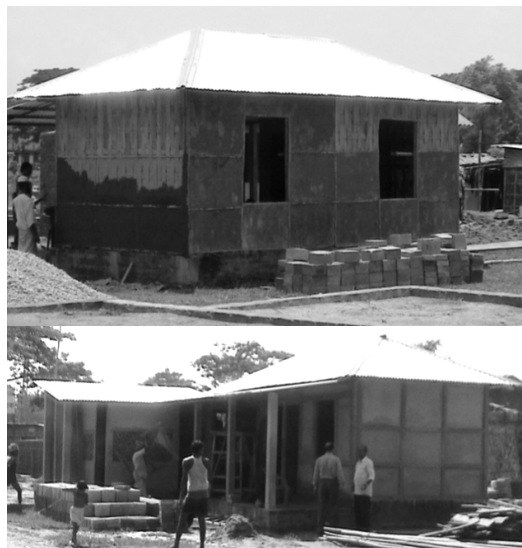
Figure 4: Prototype 4 Ekraw wall construction
