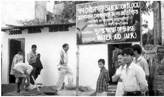
Figure 4: Community Clustered Latrines. (Source: Hanchett, S., Akhter, S., Khan, M.H., 2003)
