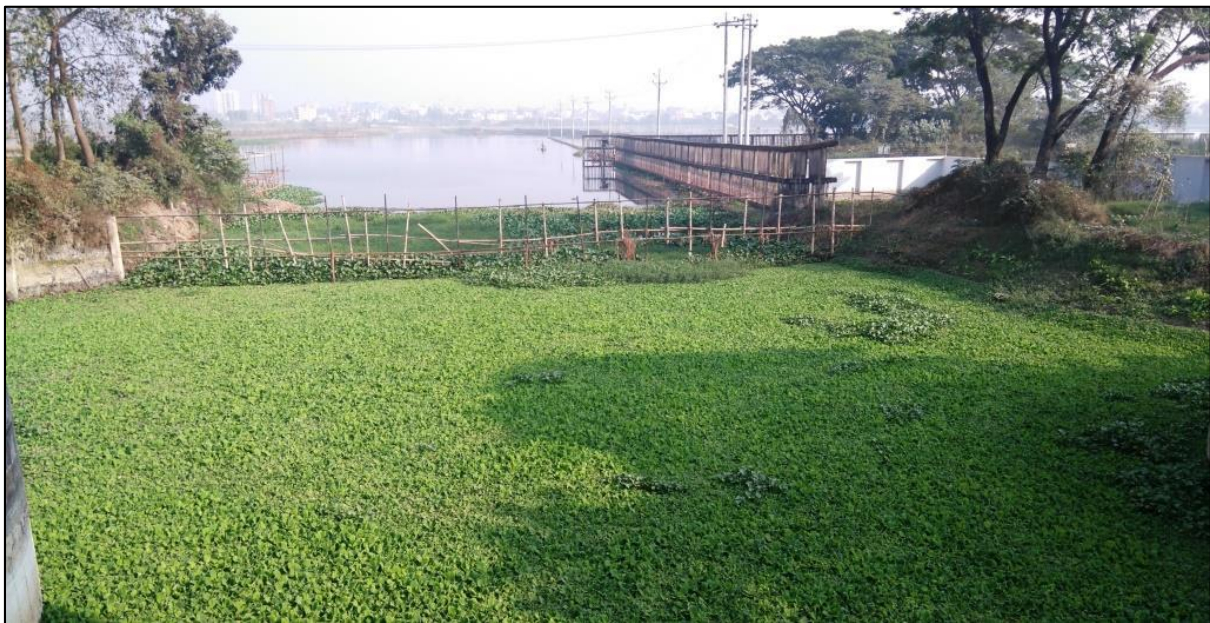
Figure 5-14: Retention pond near Goranchatbari Pump Station (River Side)
