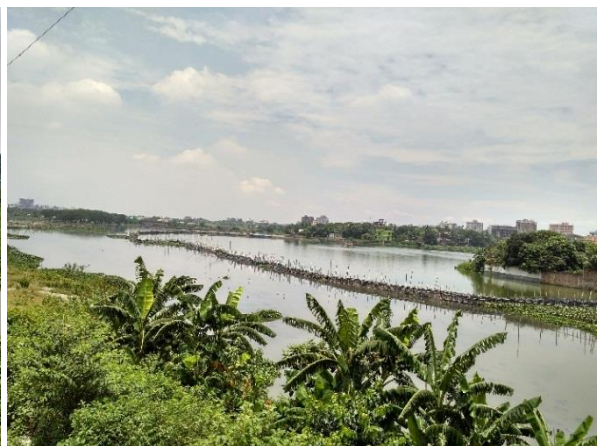
Downstream of Bridge
