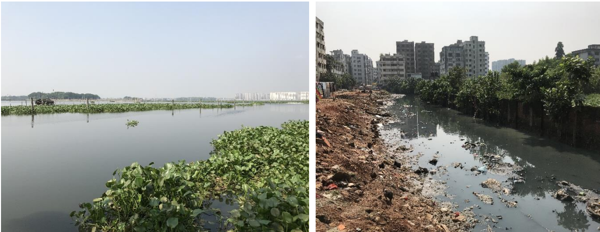
Figure 2-12: Existing Digun khal and Rupnagar Khal
