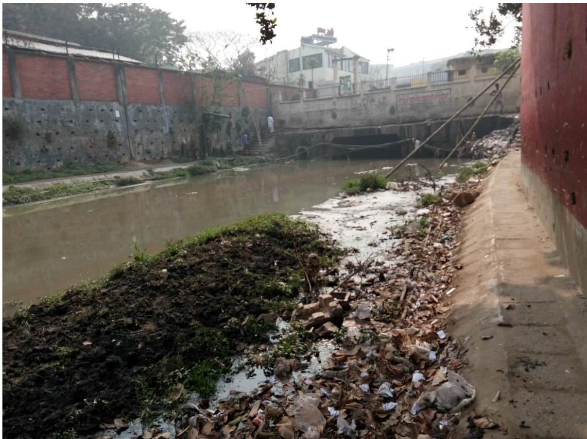
Figure 2-38: Conversion of khals into pipe drain at the mouth of Ibrahimpur Khal
