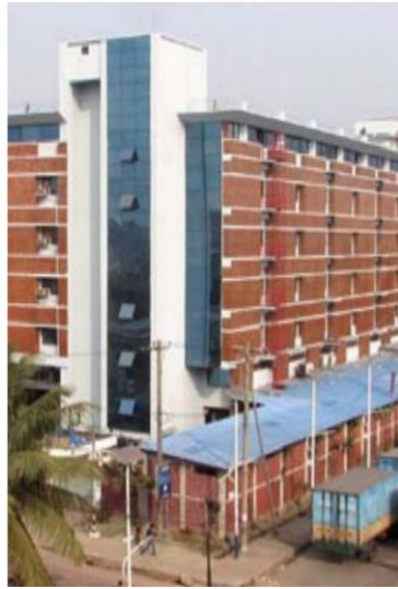
(a) Section Seven Ltd., Chattogram Height: 30 m Lat: 22.2877058 Long: 91.7750588
